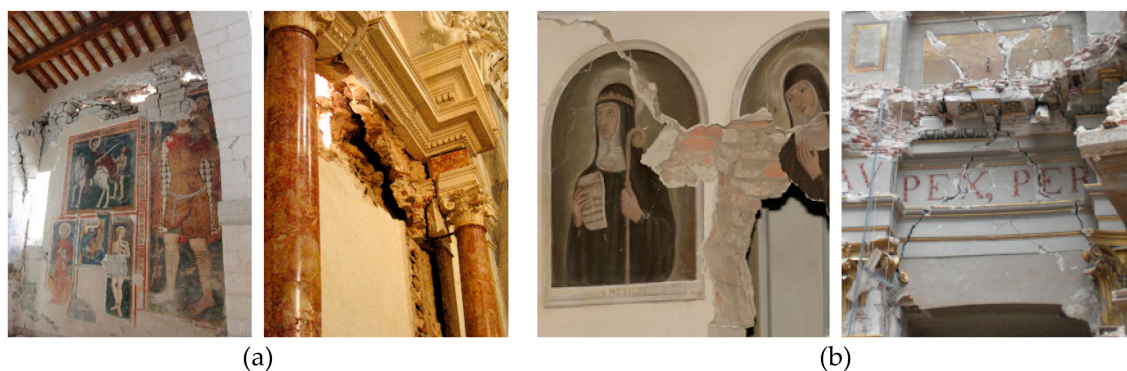
Figure 1. Examples of damage of artworks due to out-of-plane (a) and in-plane (b) mechanisms for frescoes and stuccoes.
